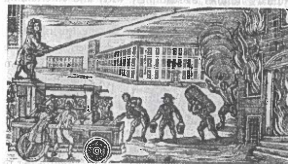
London firefighters, c. 1720. The machine is filled by hand at the front as the pumping mechanism is operated at the sides.
