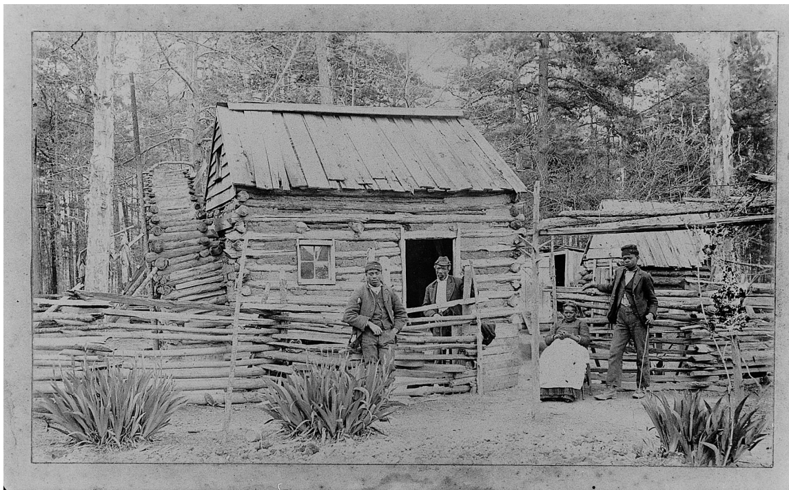
Fig. 11. An example of a one-room log cabin with a half-story above and a wooden chimney, ca. 1900. (Virginia Historical Society.)
