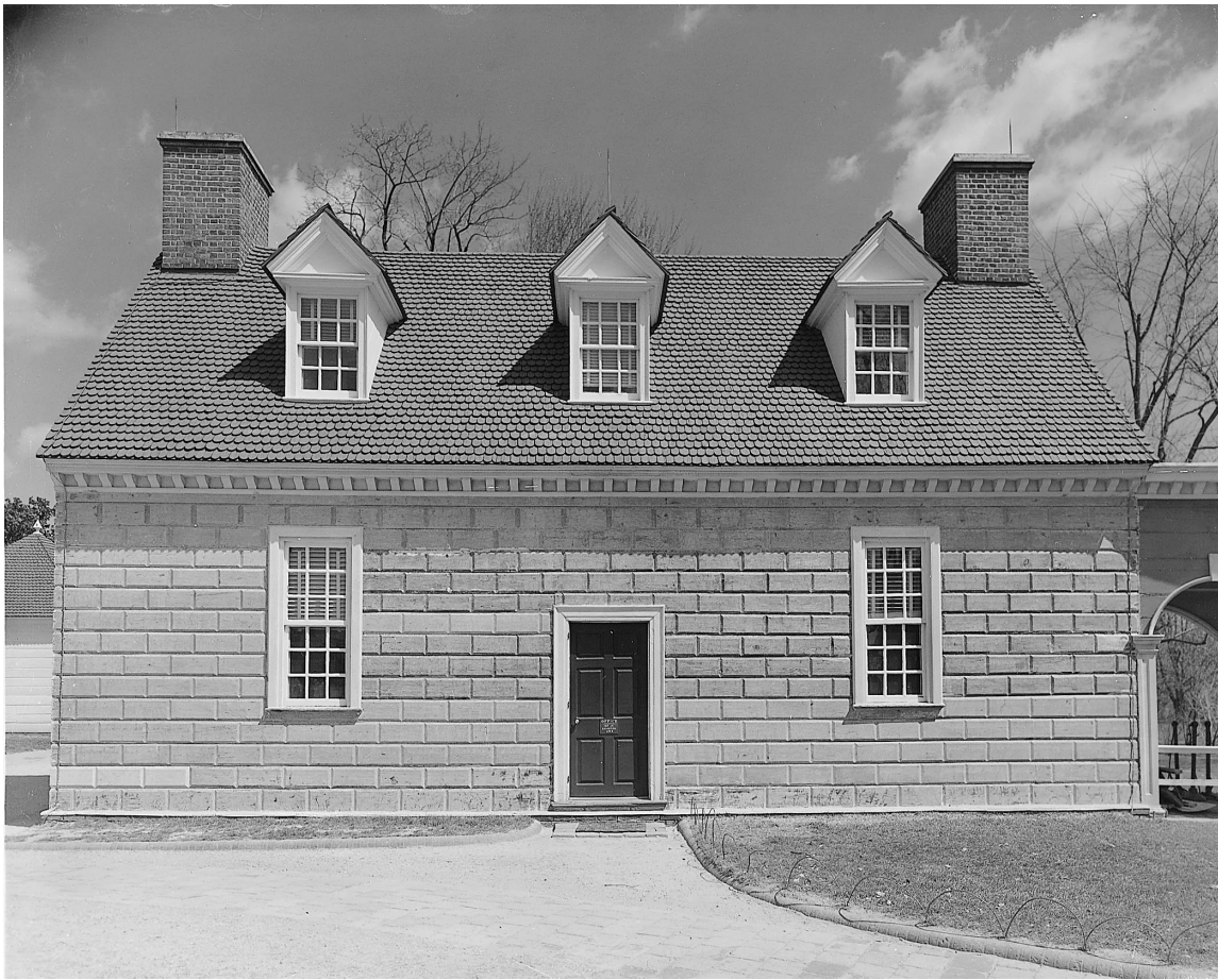
Fig. 12. Servants' Hall at Mount Vernon, 1775. (Mount Vernon Ladies' Association.) The photograph was taken during the process of repainting in 1961.
